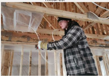
A student working for Pro North Heating and building an intake vent using a tinner's hammer, for a commercial heater.
